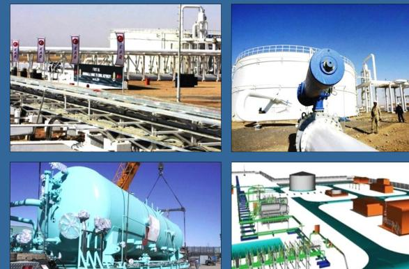
**Underground Gas Pipelines** 20 inch 68.6 km, 24 inch 32 km **Aboveground Crude Oil Pipelines** Wells - Stations (6 inch 55 km) **Underground Water Pipelines** (4-8 inch) **Block Valve Stations** 2 x Crude Oil Pipeline 2 x Gas Pipeline 2 x Temporary Water Pigging Station
